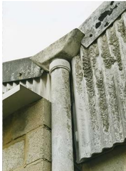
Asbestos cement downpipe, hopper and profile sheet
