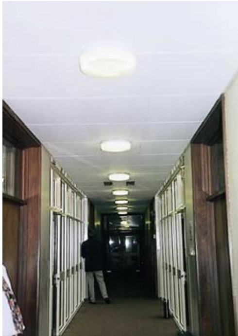
Suspended Asbestos Insulating Council tiles in a corridor
